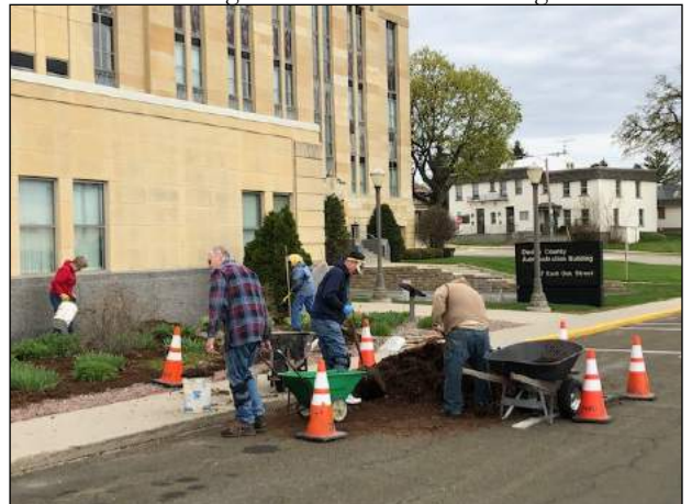
Working at Administration Building
